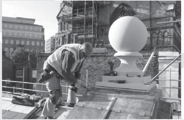
Dave Smith (Smith's Roofing), puts on the lead flashing.
