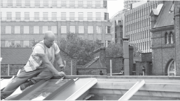
John Llewellyn, Re-glazing the roof
