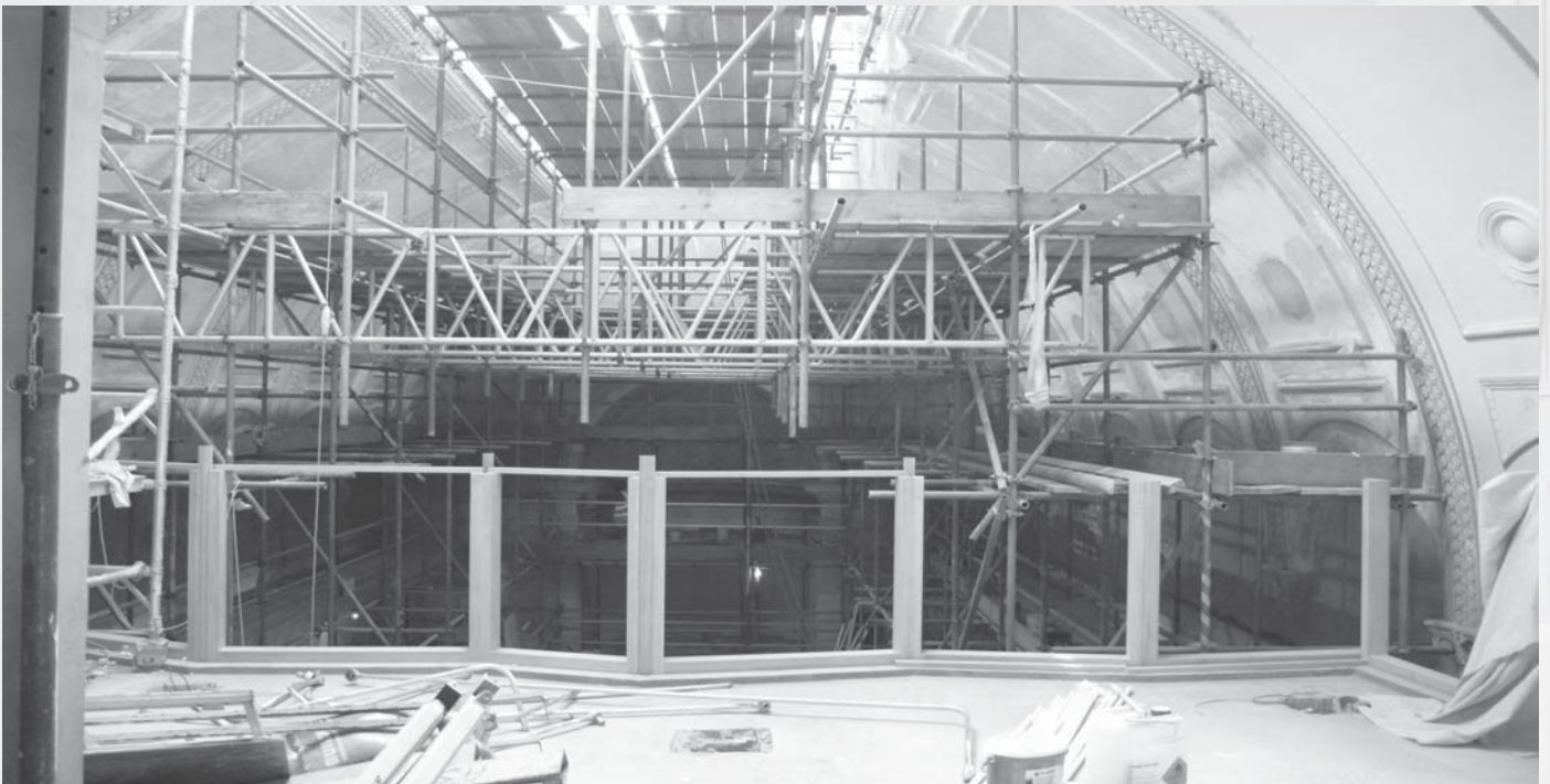
View from the gallery onto massive scaffolding
