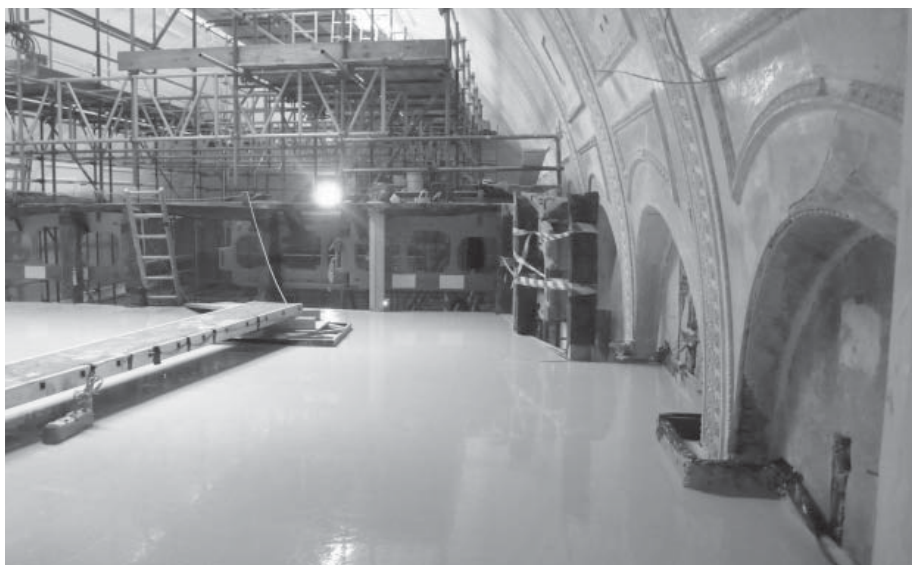
Freshly laid screed floor on gallery
