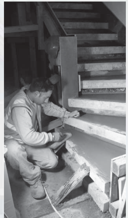
Finishing the elegant new staircase
