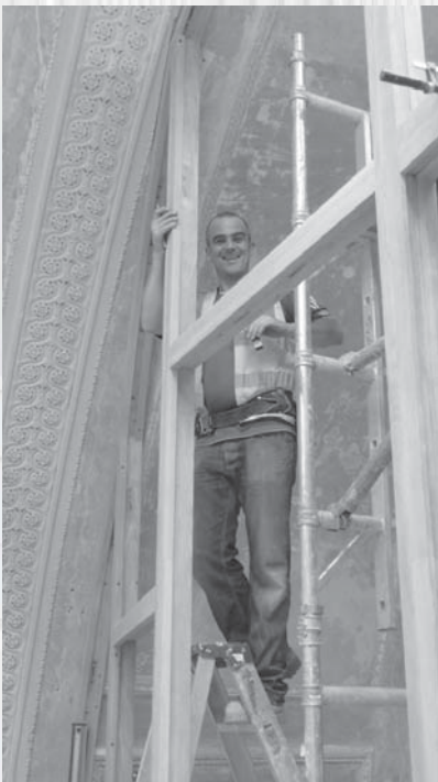
Robert Badder, Carpenter (Saltash), installing the frame
