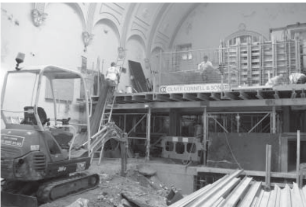
Shuttering for lift shaft on office floor is being erected
