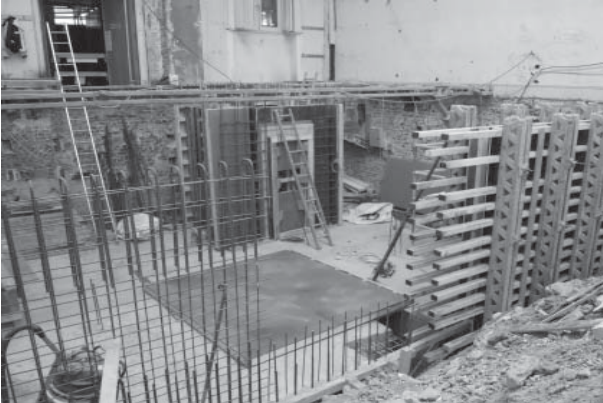
Building the shuttering for the retaining walls in the basement
