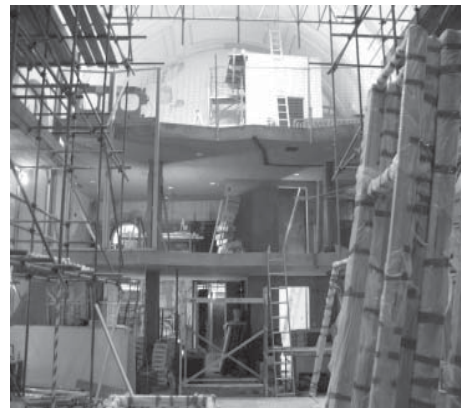
Wooden frames ready to be erected
