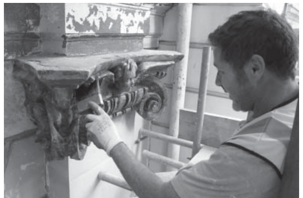
Tony Flood (APC) puts on a sealer on the external facade
