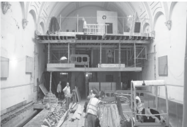
All floors and lift shaft built
