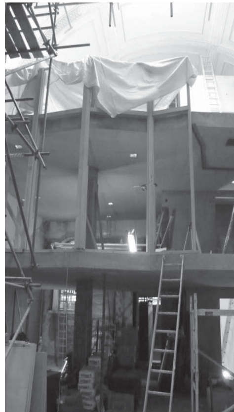
First wooden frames erected to form inner façade
