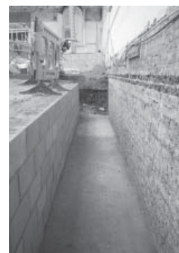
Building the service trenches (for air circulation, extracting kitchen air)
