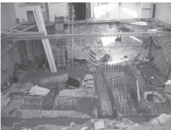
Commencement of steel fixing on 50mm of concrete blinding floor.
