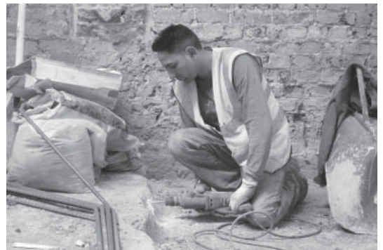
Gurmeet Singh, Steel fixer, Oliver Connell, specialists for reinforce concrete
