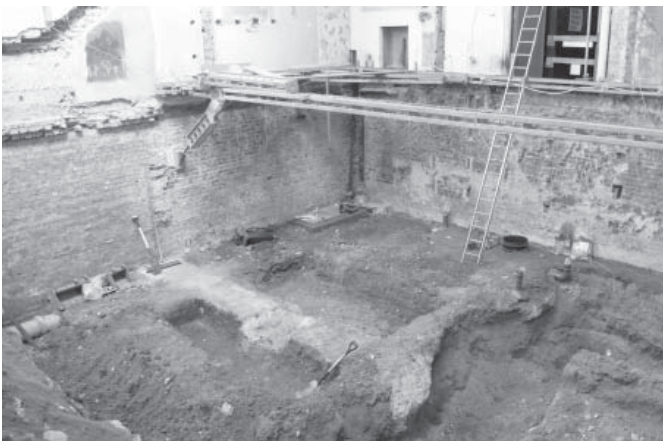
Excavation complete with foundations for columns and lift.
