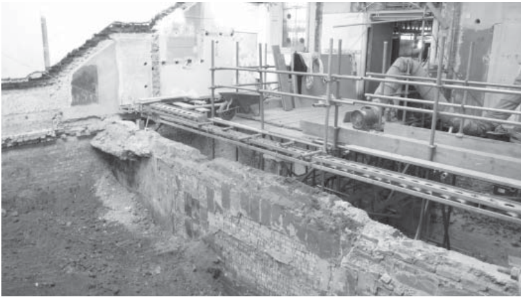
Excavation before demolition of retaining wall.
