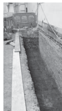
Building the service trenches (for air circulation, extracting kitchen air)
