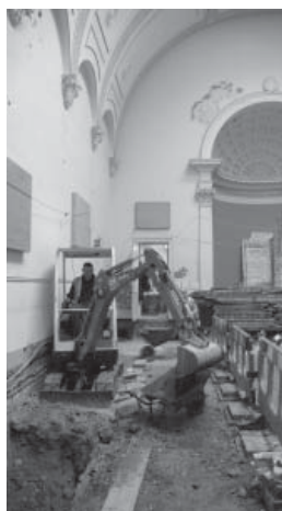
Building the service trenches (for air circulation, extracting kitchen air)
